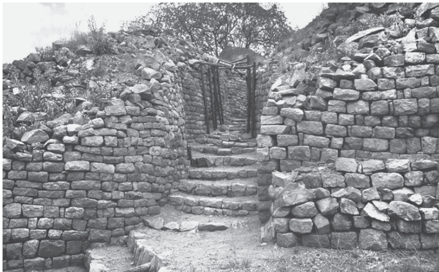
Figure 5.7 Southern Passage shored up with iron bars
